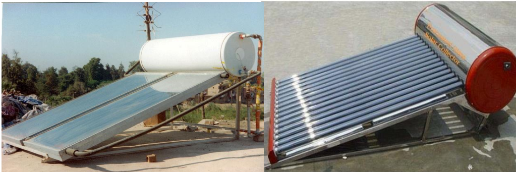
Solar water heaters in Lagos
