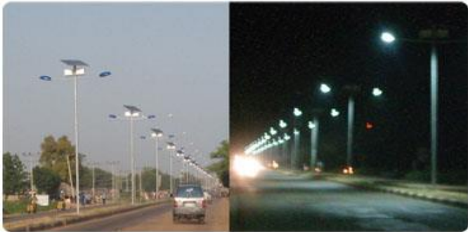
Street lights in Jos
