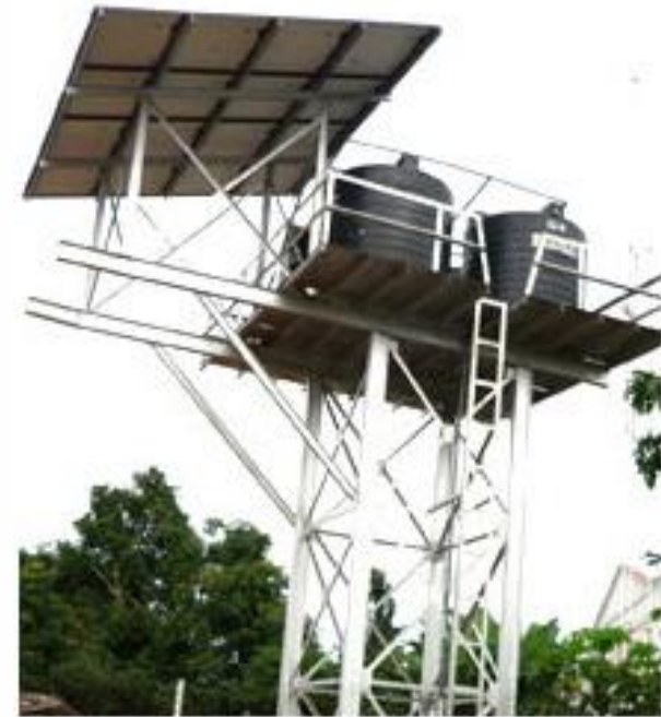
Solar water pumping in Katsina – Green wall project
